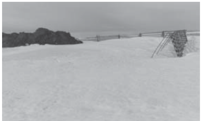
Snow fences and berms ensure maximum snow build-up
