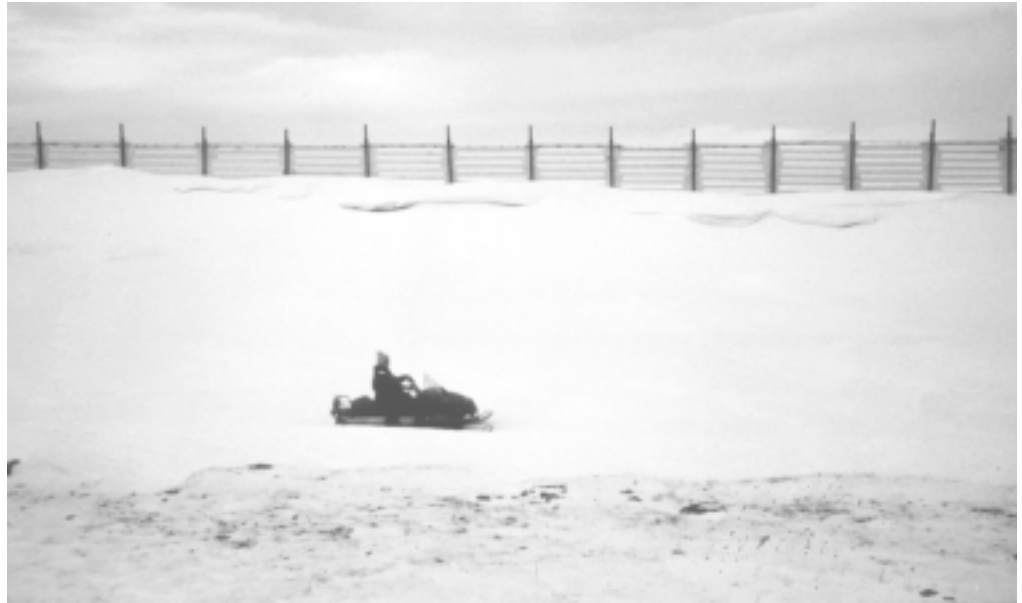
Snow fences are very effective at catching and storing wind-blown snow in dugouts
