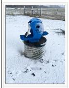
"We installed the first one eight years ago and used a backhee to dig deep enough to have water coming into the hole, and put a culvert into that hole—about is feet down—then put gravel around it. We'd drilled holes around the bottom end of the culvert to allow water to come into it," Alvin Lusk explains. [Photo courtsy Alvin Lusk.]
