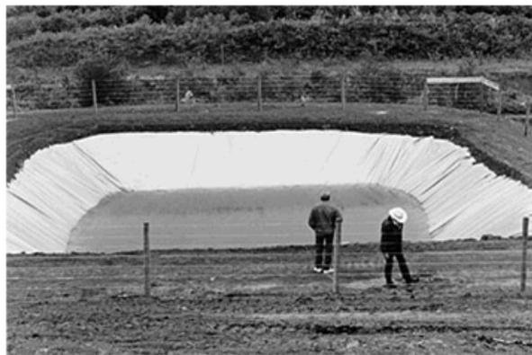
Figure 2. Elevated earthen reservoir with woven polyethylene liner
